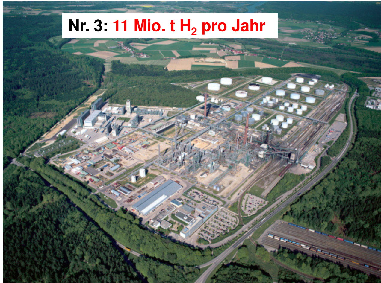
Refinery Burghausen, Germany (courtesy of Linde Eng., Germany)
